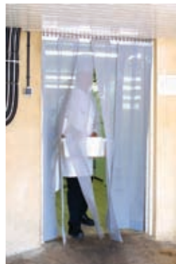
Cold store with PVC strip curtain
