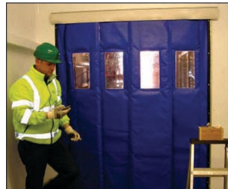
Cold store with insulated strip curtain
